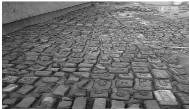
Figure17: Water proofing process
