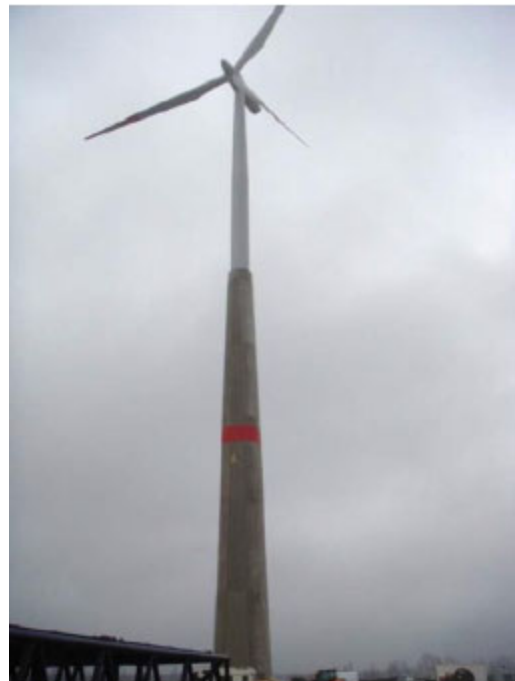
Fig. 4.13: Steel hybrid tower
