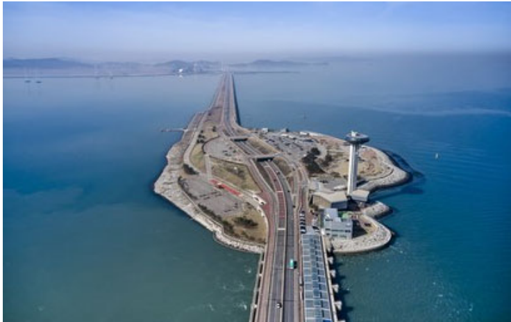
Fig 7.2: Sihwa Lake Tidal Power Station, South Korea (Courtesy: Shutterstock)
