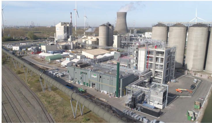
Fig 6.6: Waste-based biodiesel power plant in Belgium.
