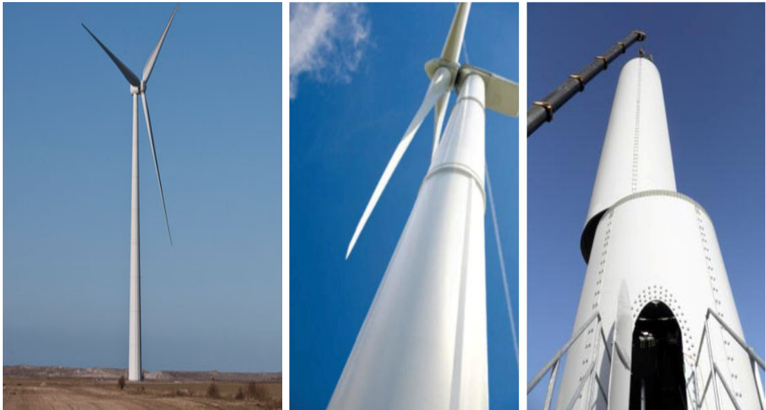
Fig. 4.11 Tubular steel tower
