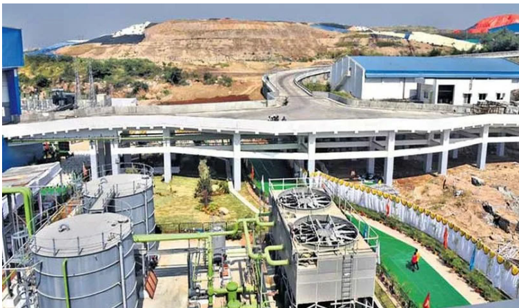
Fig 6.5: A 20 MW municipal waste to energy plant at Jawahar Nagar, Hyderabad.
