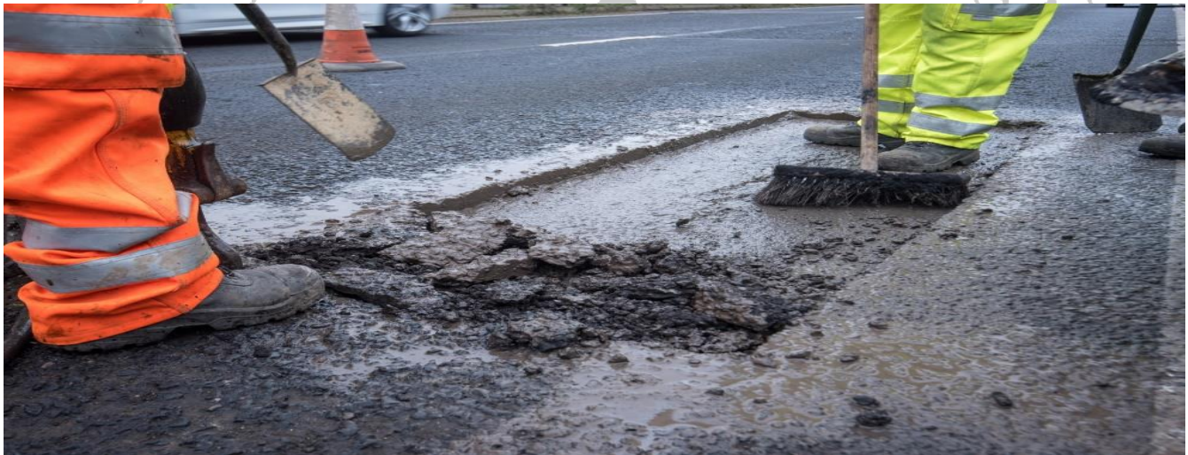
Figure 15.2: Road Repair Work
