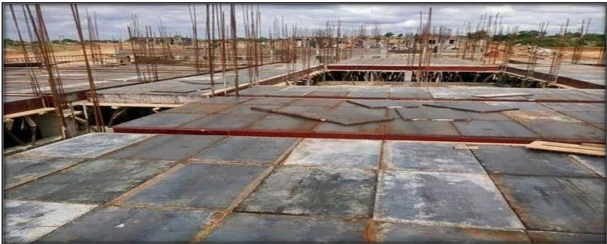
Figure 12.3: centering work
