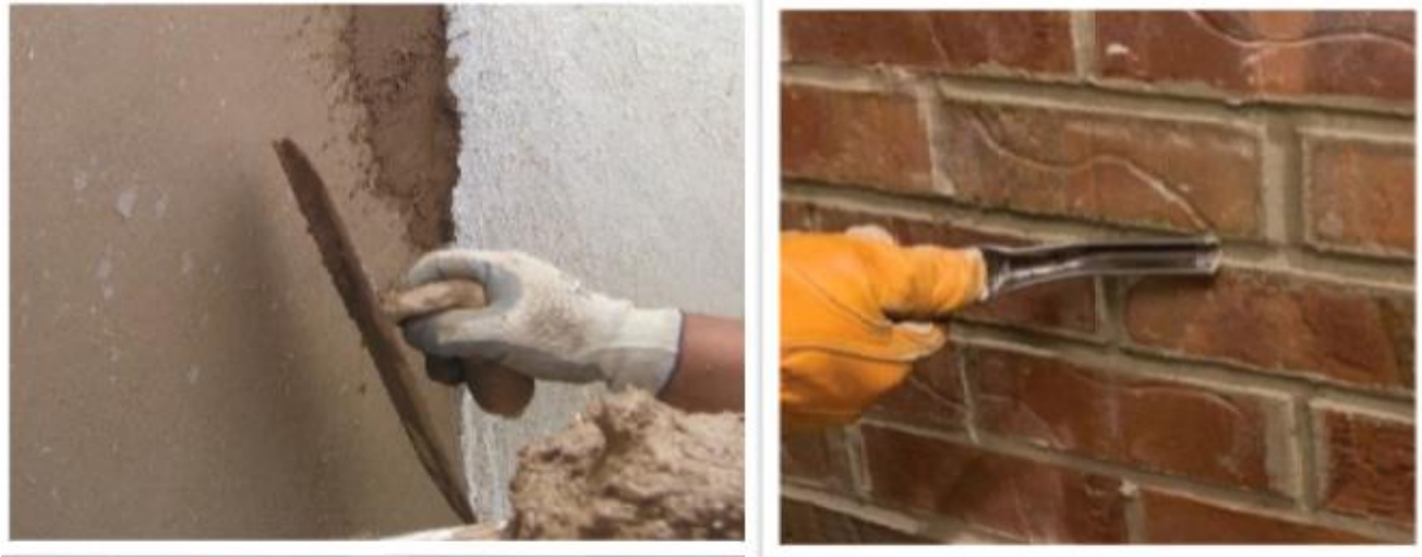
Figure 16.1: plastering and Pointing
